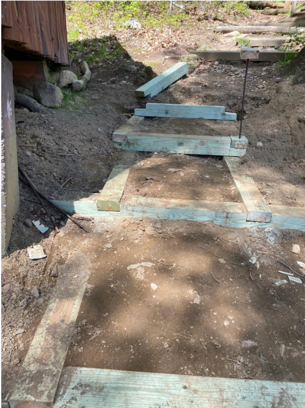
NEW STEPS TO BEACON WERE COMPLETED AND HELD UP TO THE FLOODING
